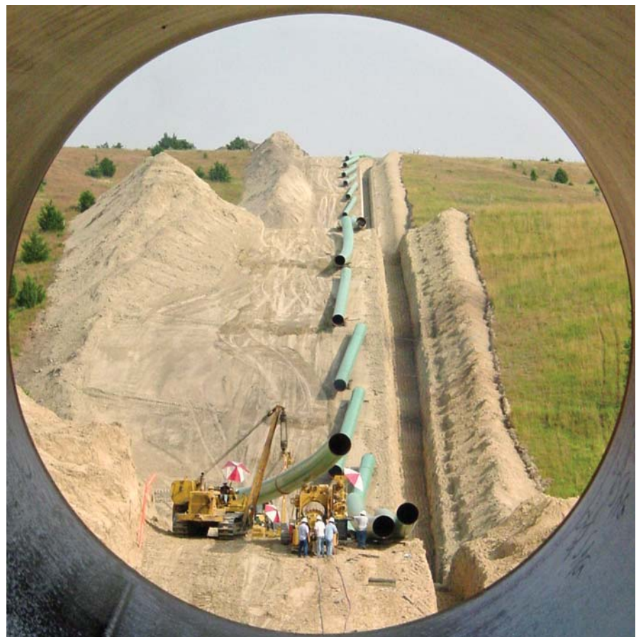
REX West Construction photo by Butch Stovall
